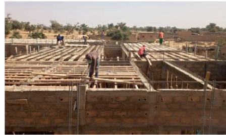
January 23, 2021—Admin. building
