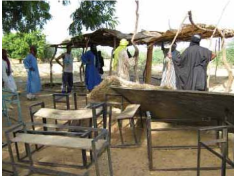
Parents building hangar
